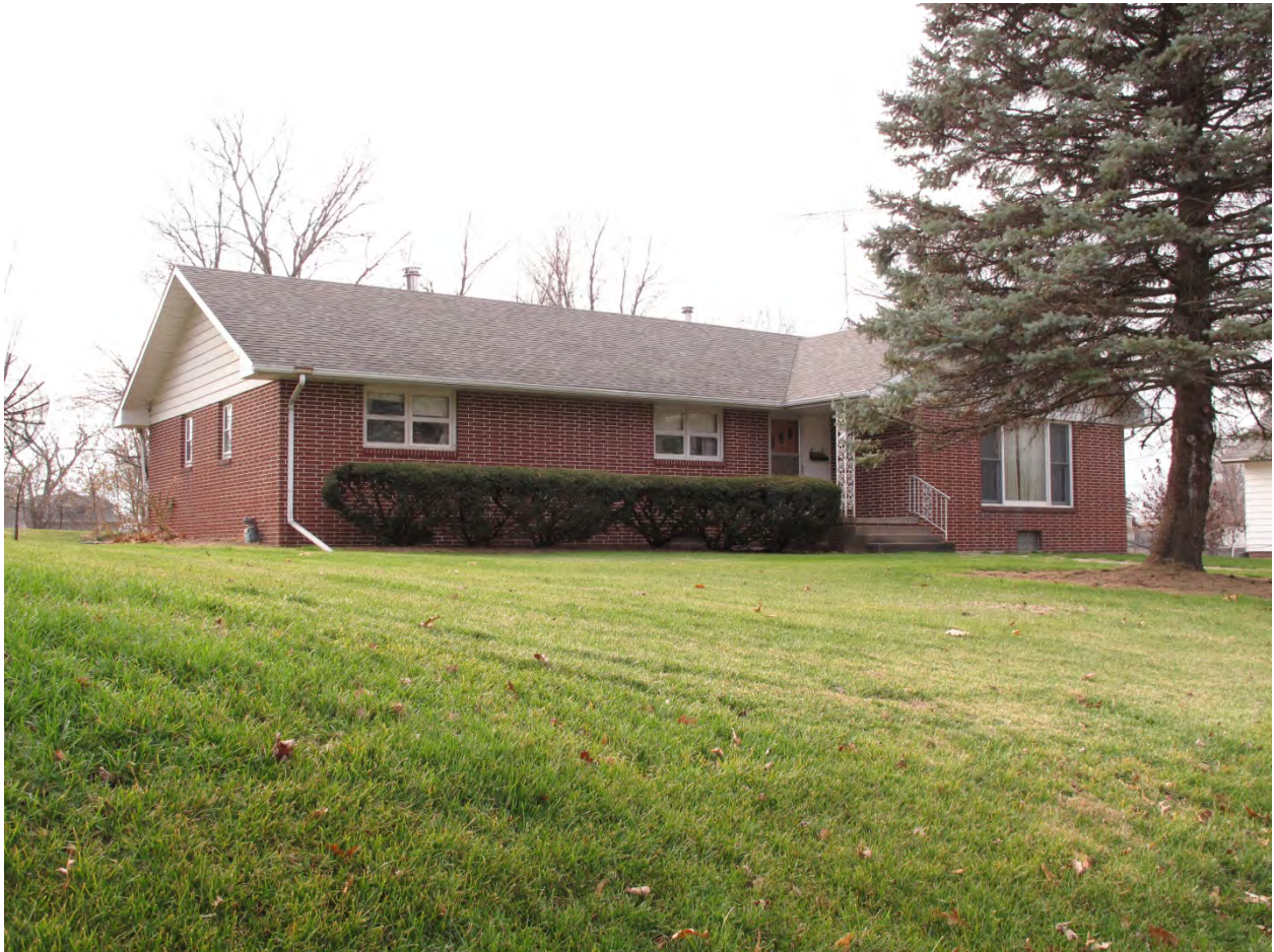
Fair Oaks\Photos\IMG_0003.JPG - R.L. McCarley, November 2012
